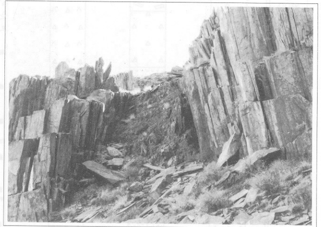
C.1d: Layering-parallel fracture cleavage with a vertical to steep northeast dip in rhyolite flows and ash-flow tuff of the HFF. The ash-flow tuff ( \approx 3 m thick) exhibits a more weathered and fractured appearance due to its less competent nature. Southern locality of the HFF. (Map - Appendix I).
